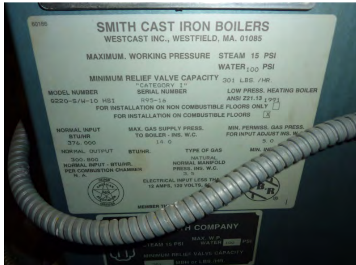
Typical cast iron boiler is shown to be replaced mid-plan.
