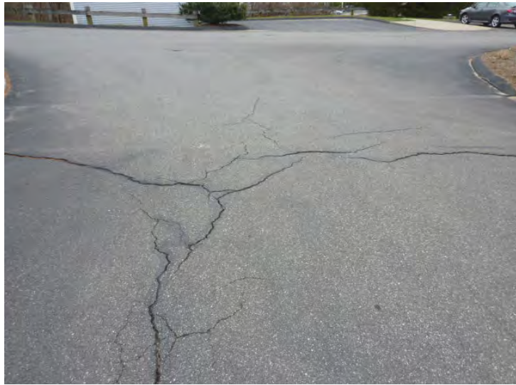
Asphalt paving exhibits historic crack sealing. Shown is typical new cracking site-wide that has not been sealed and will lead to sub-base failure.
