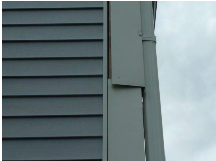
Typical aluminum cladding failure at trim.
