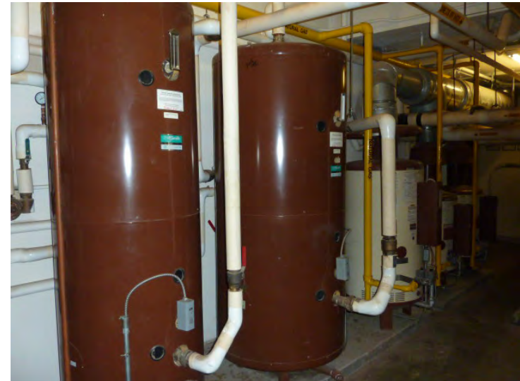
Typical hot water storage tanks and hot water boilers behind are shown to be replaced mid-plan.
