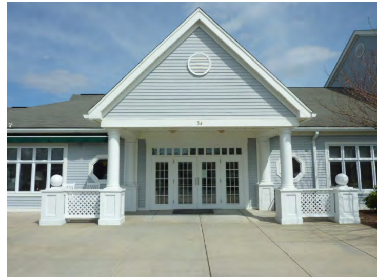
Typical concrete walks and paving at front entrance is in good condition. Storefront is exhibiting serious signs of distress.
