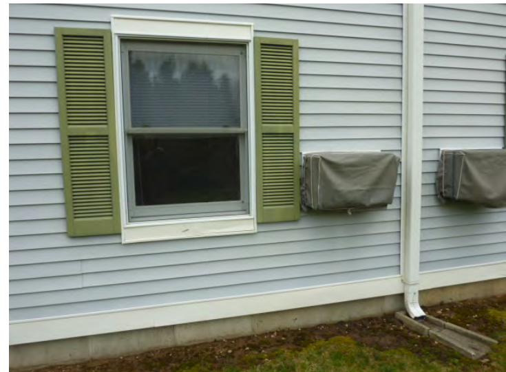
Typical worn and mottled vinyl siding and trim, faded vinyl shutters and deteriorating screen mesh.
