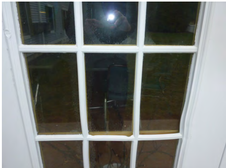
Insulating glass at storefronts has fogged due to failed seals, and the mullions and muntins are warped.
