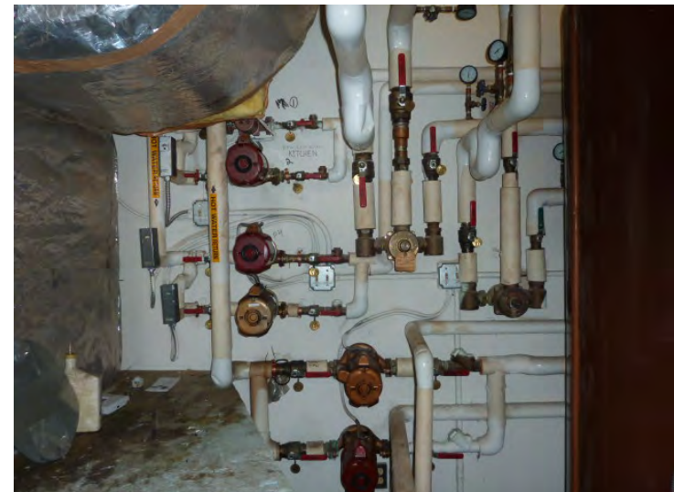
Circulating pumps are shown to be replaced late in the plan.
