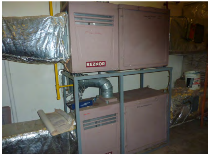
Reznor duct furnaces are shown to be replaced early in the plan.
