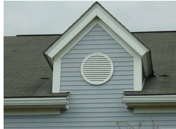
Typical raised shingles at roof ends of gable eaves is reportedly the source of localized leaking.
